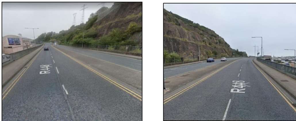
Plate 5.4, 5.5 Views of R448 Dock Road looking west and east respectively
